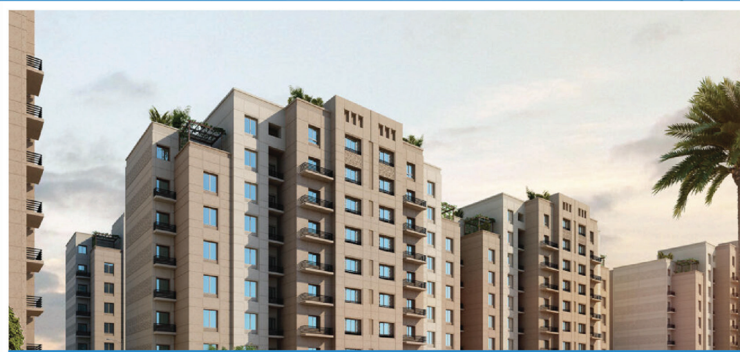
Bouvardia View - Jeddah -
